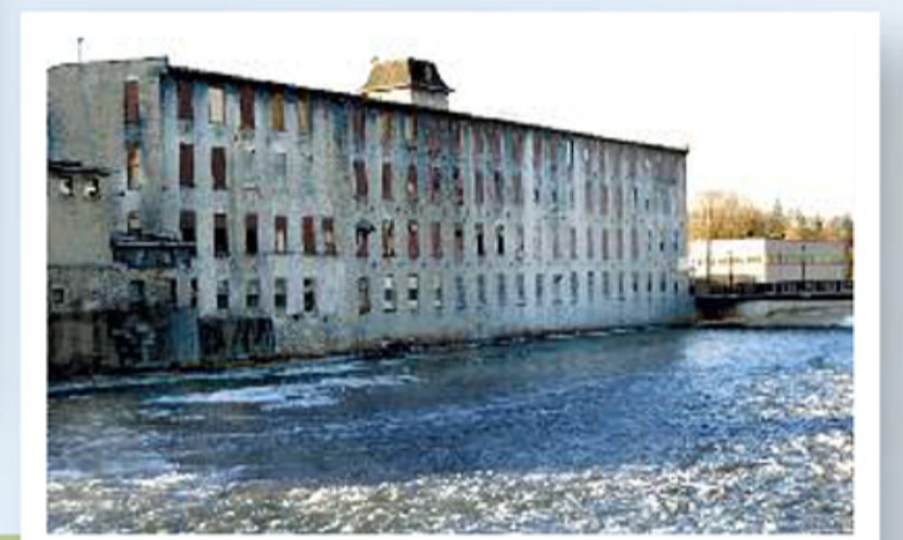
▲ American Standard—one of Hespeler's main businesses along the Speed River—started up in 1847. Today, this historic building is being converted into luxury condominiums. American Standard factory in Hespeler.
